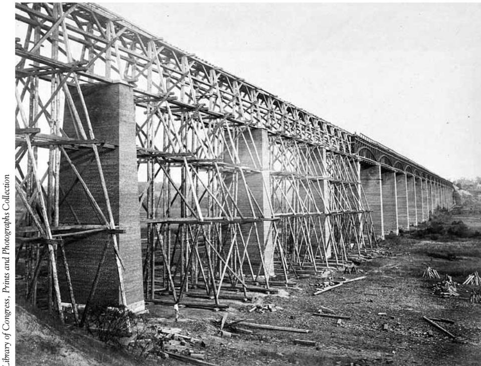
**High Bridge, ca. 1865. Photograph by Timothy H. O'Sullivan, following the Battle of High Bridge, showing the reconstruction of four spans damaged during the battle.**
