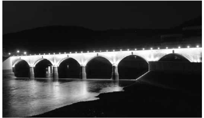
The PRR's Conemaugh River Viaduct, Johnstown, Pa., lit at night.
