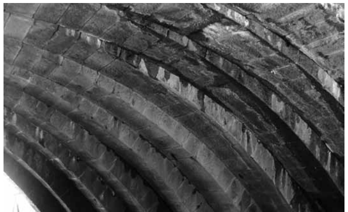
The Johnstown Bridge's ribbed arches.
