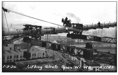
This view, taken Jan. 3, 1936, shows workers on the west span of the Bay Bridge, high above the San Francisco waterfront. The caption indicates that the workers are lifting struts into place between the main cables in preparation of constructing the deck. The SIA Samuel Knight Chapter toured the Bay Bridge in May.
