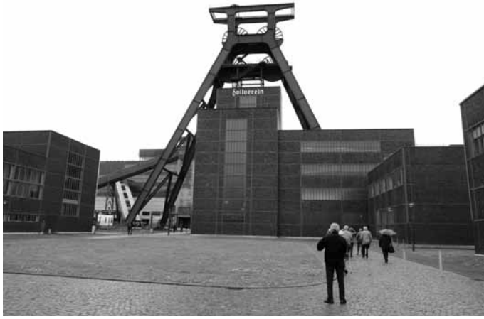
Head frame and museum at Shaft 12, the Zeche Zollverein colliery.
