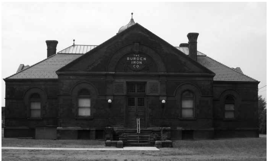
Burden Iron Works.
