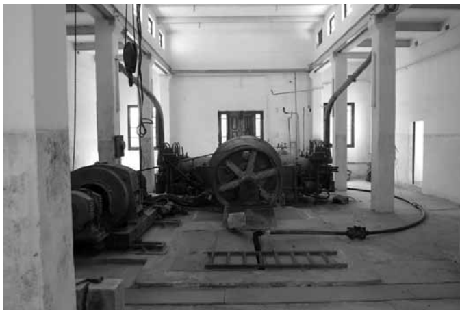
Volunteers recently restored to operating condition the engine at the 1935 Wied il-Ghasel pumping station.
