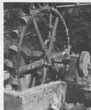
Rare alternating-bucket impulse turbine direct-connected to a cross-compound air compressor, c1890. Salmon Creek Falls.
